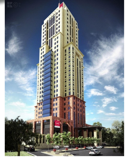
UAP Building Upperhill
