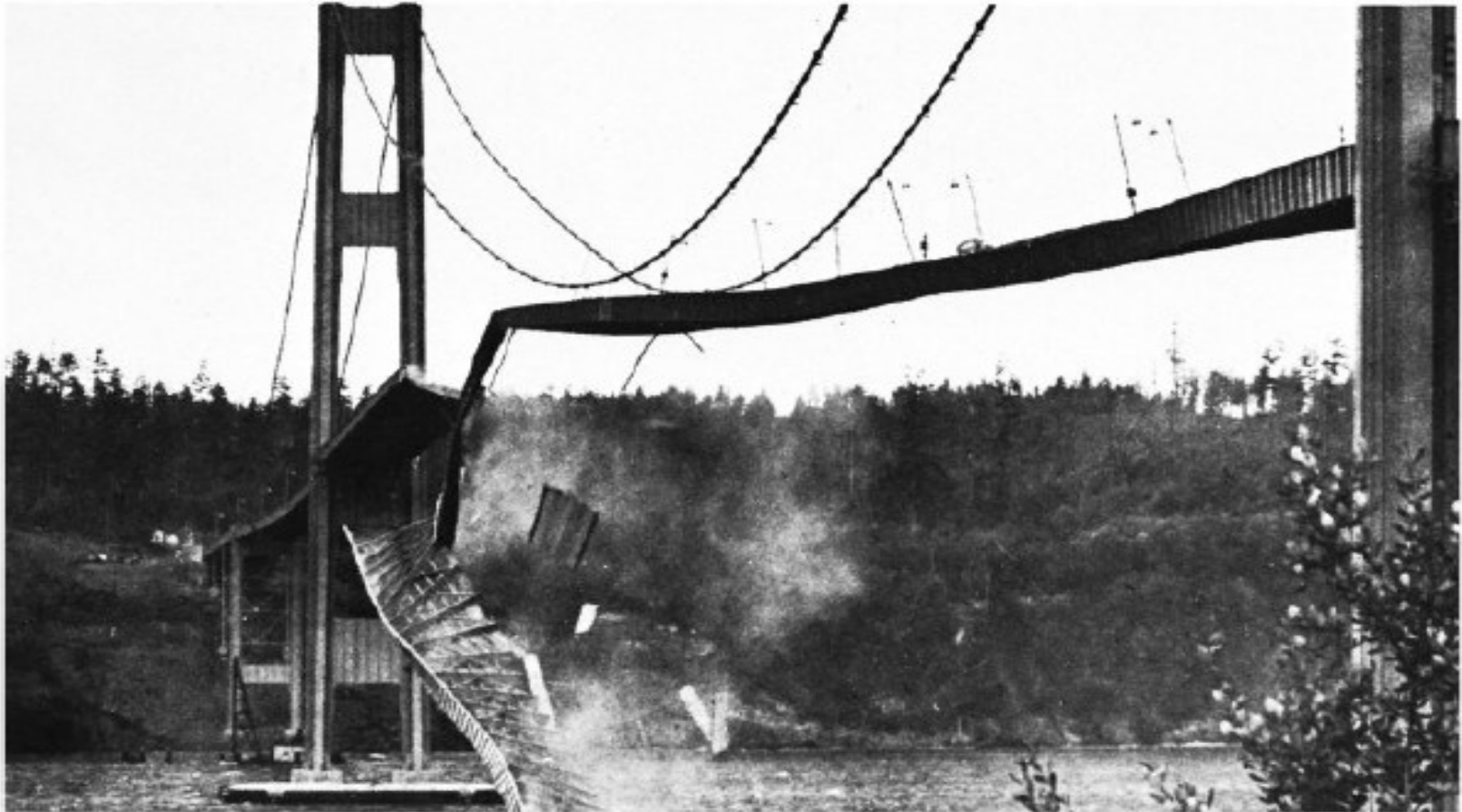
FIGURE 1.7 Tacoma Narrows bridge during wind-induced vibration. The bridge opened on July 1, 1940, and collapsed on November 7, 1940. (Farquharson photo, Historical Photography Collection, University of Washington Libraries.)
