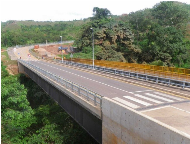
Rusumo International Bridge at the border of Rwanda and Tanzania (Completion, Jan 2015)
