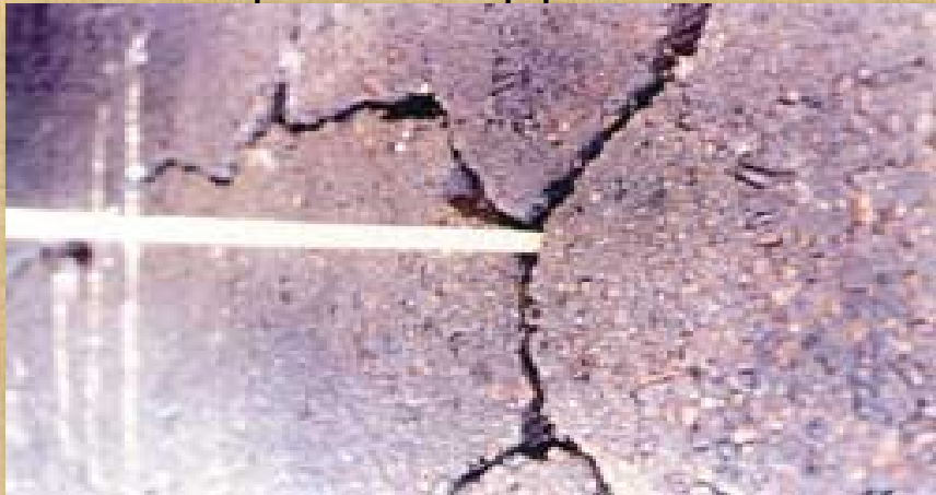
Alkali aggregate reaction
