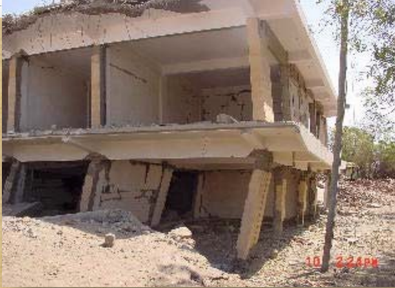
RC building collapsed in a side sway mechanism.(India)
