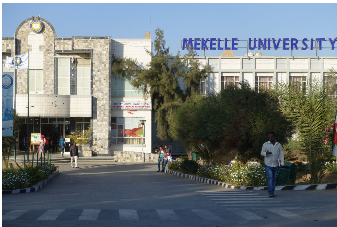
Figure 1 Mekelle University (Ayder) Hospital, Mekelle.
