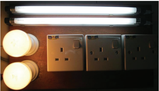
Figure 25: Appliance Board Output. Referring to previous figure, the corresponding outputs are switched ON
