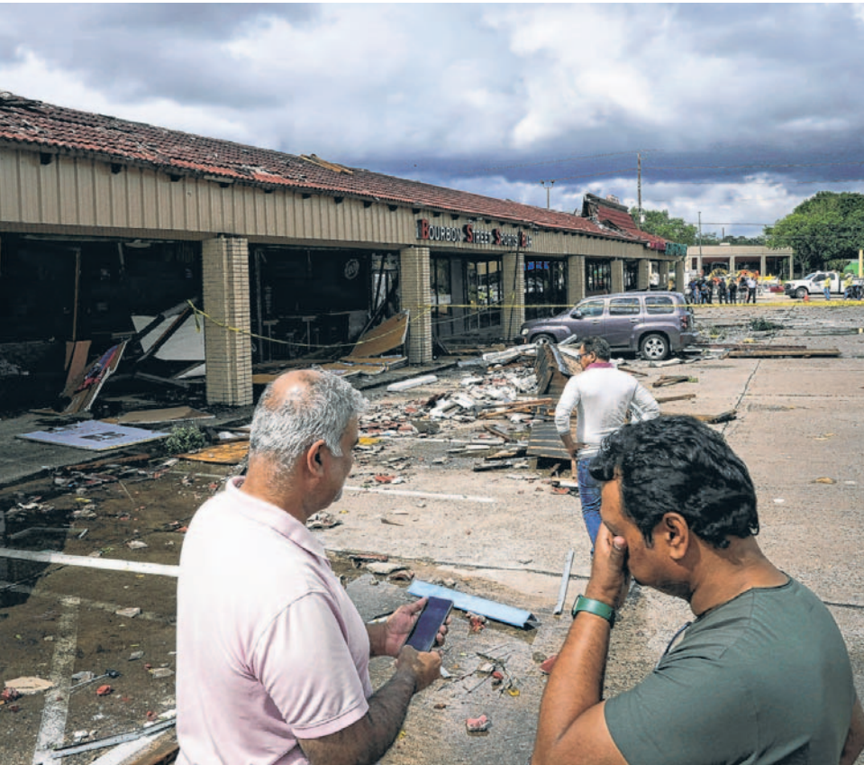
DESTRUCTION: A furniture store in Katy, Texas, was heavily damaged by a tornado. High winds tore through the South and caused flooding and road closures in some places.
