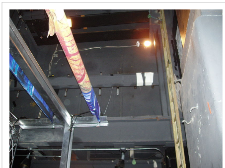
A pin-rail above stage level.
