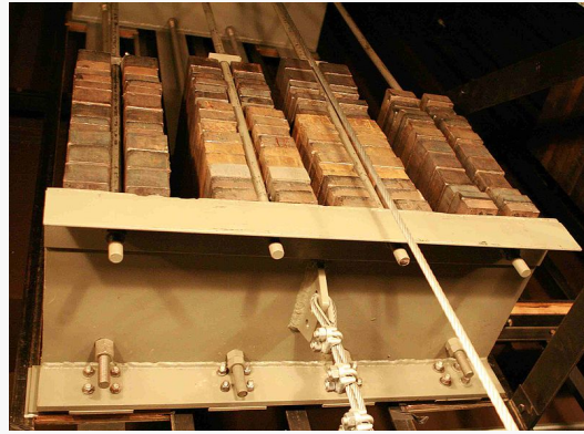
A large counterweight arbor with multiple stacks.
