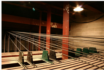
Loft blocks on a steel lattice grid.
