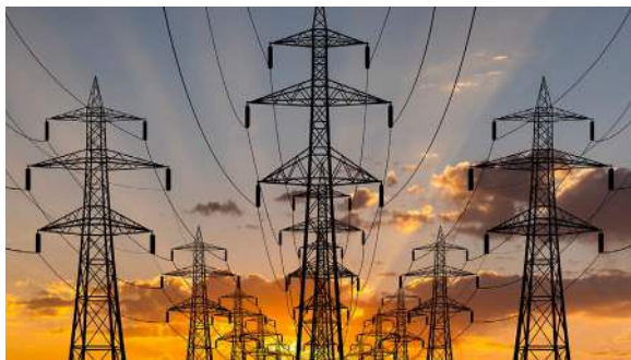
AI data centers are putting new demands on power producers.
