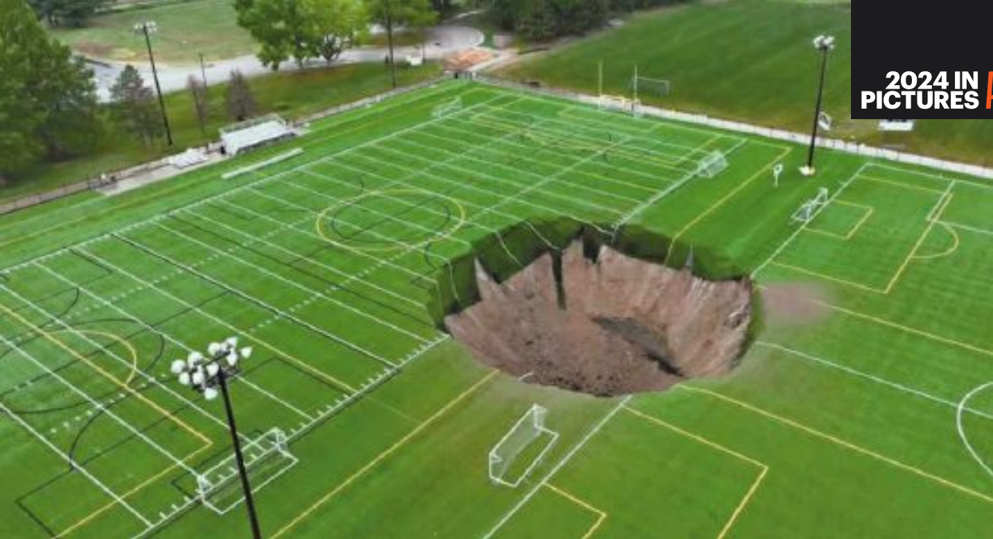
Above: a sinkhole opens up beneath an artificial grass football pitch in Alton, Illinois, on June 26. Subsidence caused by limestone mining nearby was blamed
