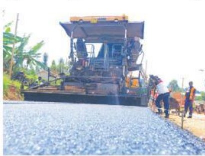
Mjinga section. Tarmacking is also ongoing around the stadium stretch while base works are complete along the Gudka-
