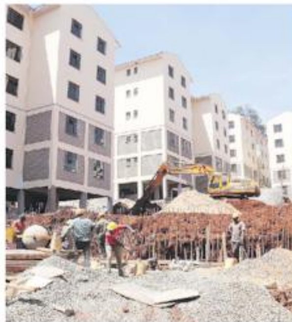
An affordable housing project for civil servants under construction by the national government in Embu County. [Joseph Muchiri, Standard]
