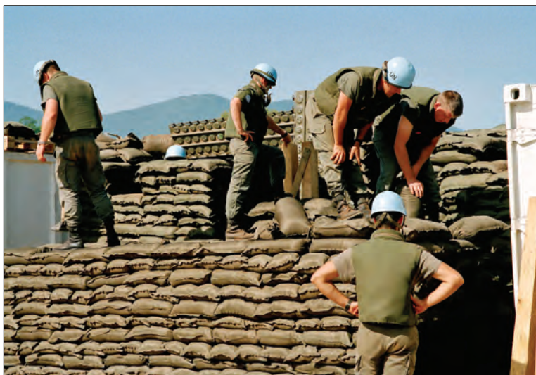
French soldiers building a sandbag bunker at Sarajevo Airport. (Source: UN Photo #121850, John Isaac)
