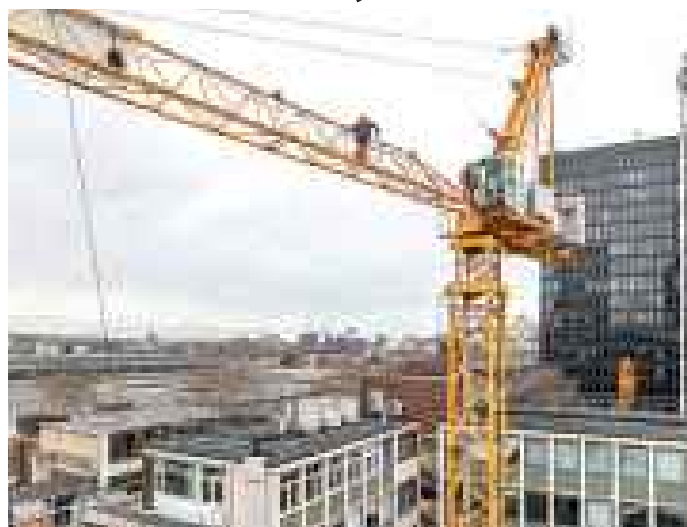
Demolition done, but what next? Tower crane in action at Euston in January 2019. The joint venture responsible for enabling works at Euston has removed this crane but carrying out more significant work on site during the lockdown is challenging as it requires workers to travel in by tube. Courtesy HS2
