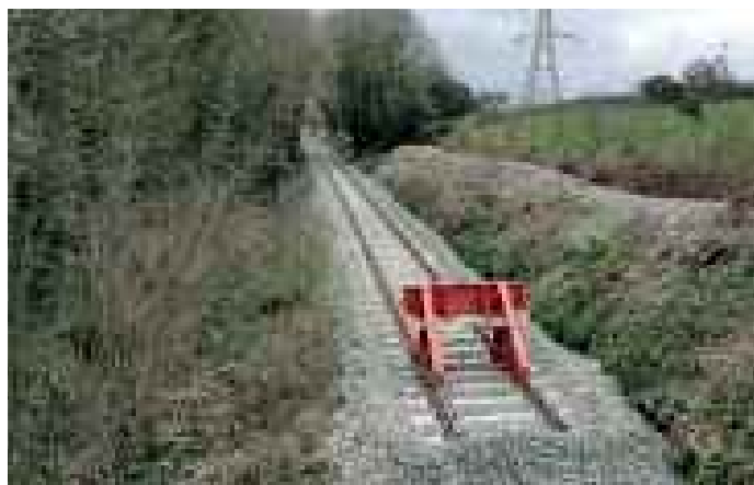
Ready for jumbo trains: an early March view of the relaid and regraded headshunt at Tytherington quarry. Richard Giles
