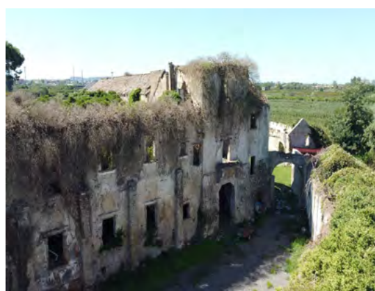
Fig.3 "Grancia di Casacelle", assonometric view with drone aerophotogrammetry by Angelo De Ciccio, internal facade of principal structure of the building in deterioration, Giugliano in Campania (NA), year 2022.
