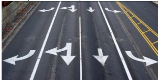
Figure 8-12: Example of Pavements arrows (AACRA)
