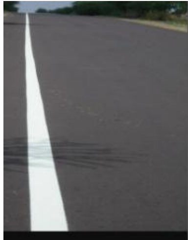
Figure 8-8: Example of Edge Lines
