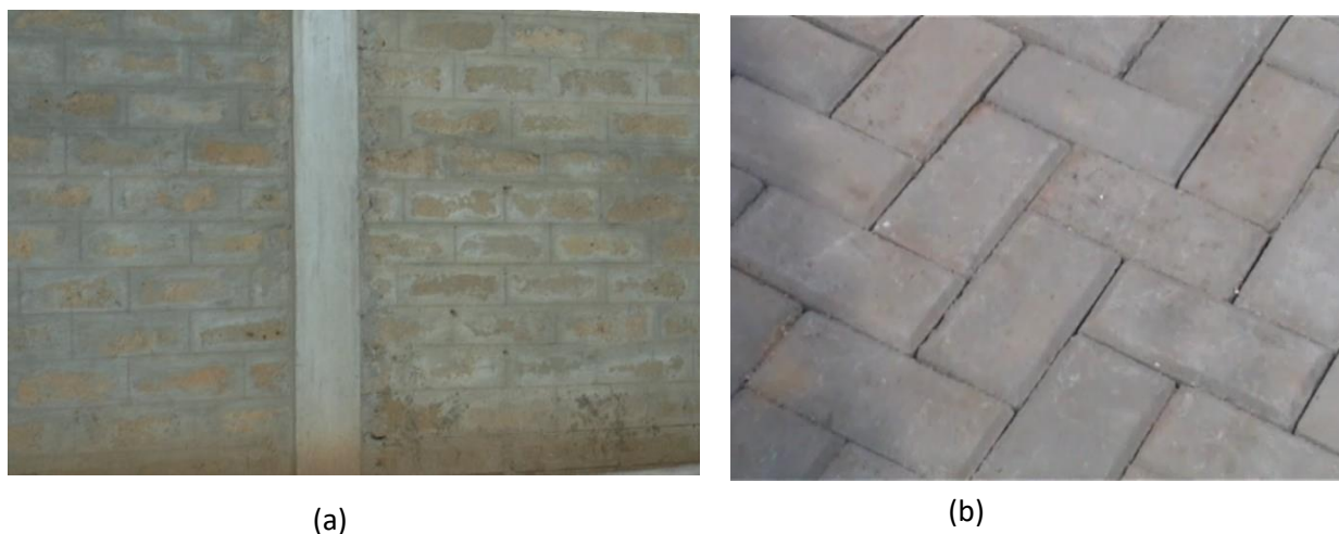
Fig. 9.2 (a) Concrete bricks and pillars for strong walls and (b) concrete pavers
