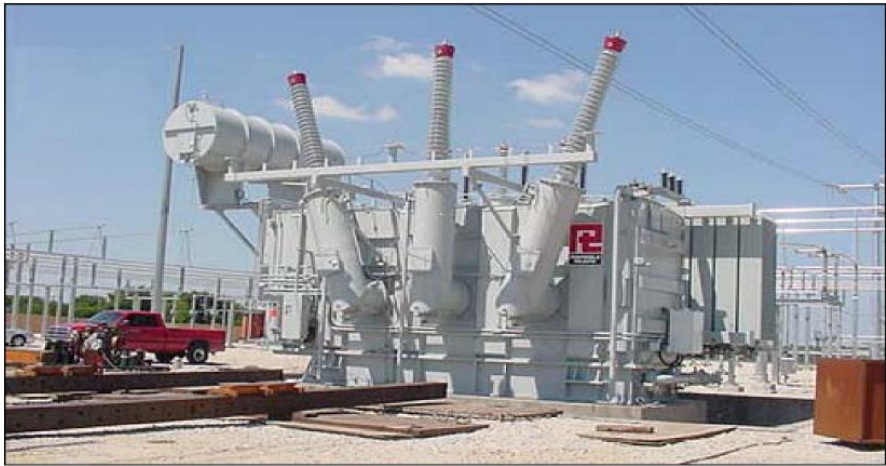
Figure 3. Installation of a 345 kV Transformer.
