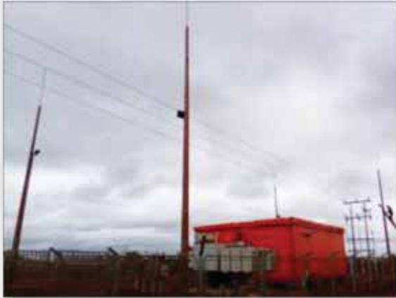
Rural Electrification Project, Niassa, Mozambique
