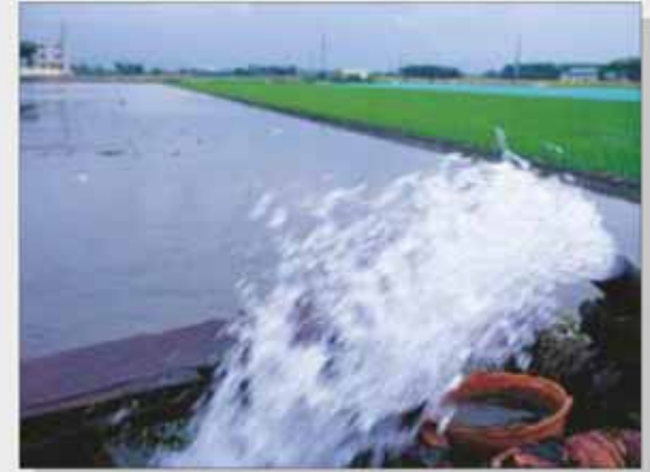
Chalinze Water Treatment Plant, Tanzania
