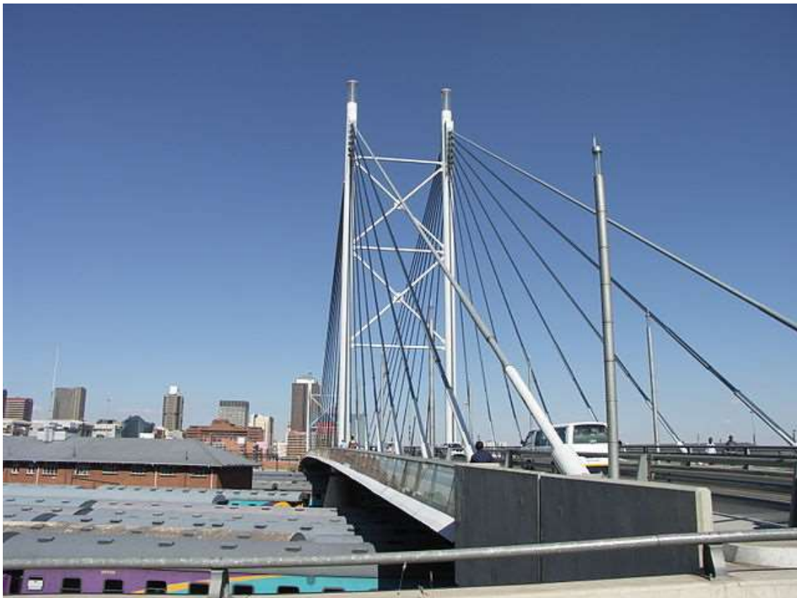
Figure 2: The Nelson Mandela Bridge
