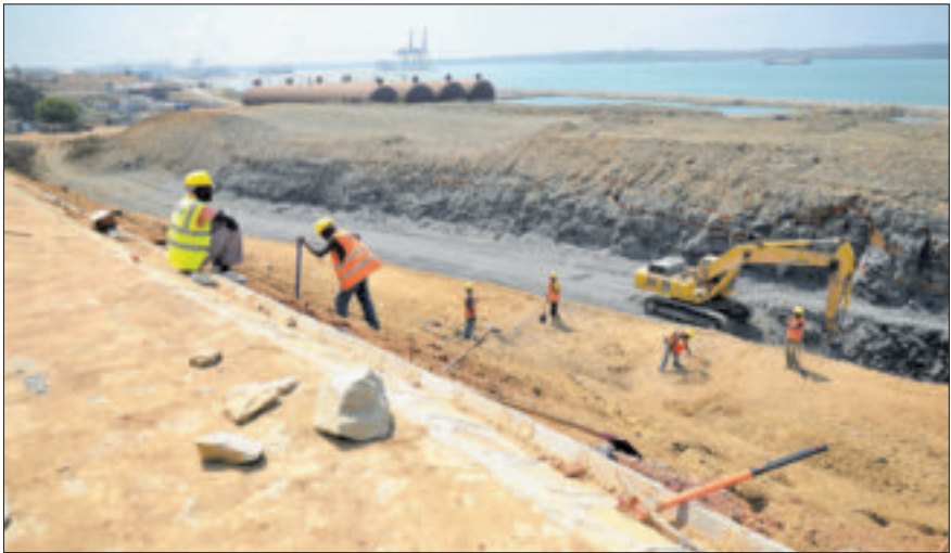
Construction of the Standard Gauge Railway terminal near Port Reitz in Mombasa on March 15, 2016. One can file a case to stop a project if it affects the environment. SALATON NJAU
