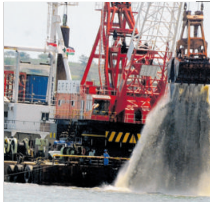
Construction of Kenya Port Authority's second container terminal began at the project funded by Japan International Co-operation Agency to the tune of
