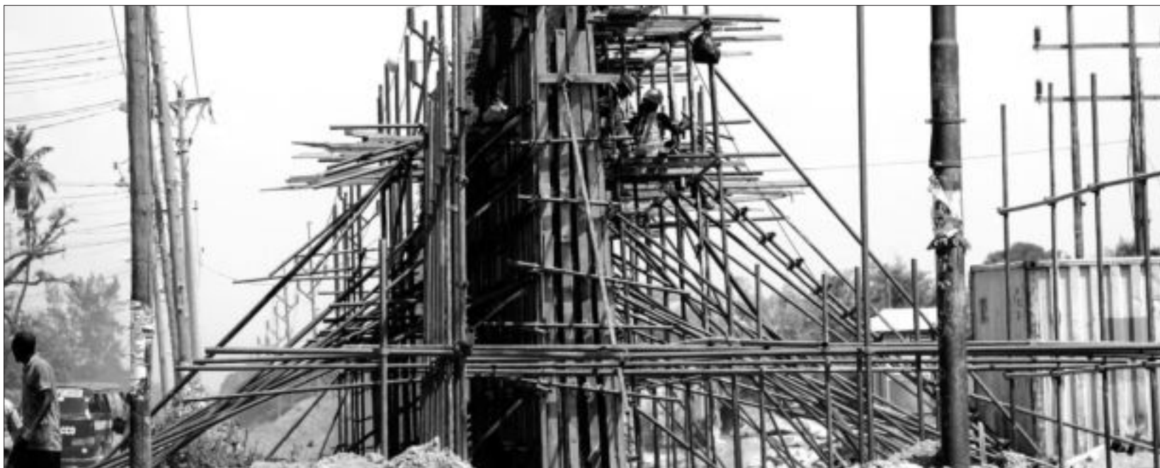
Workers constructing the Changamwe-Airport Road round-about that is part of the projects being implemented in Mombasa to ease traffic congestion. LABAN WALLOGA
