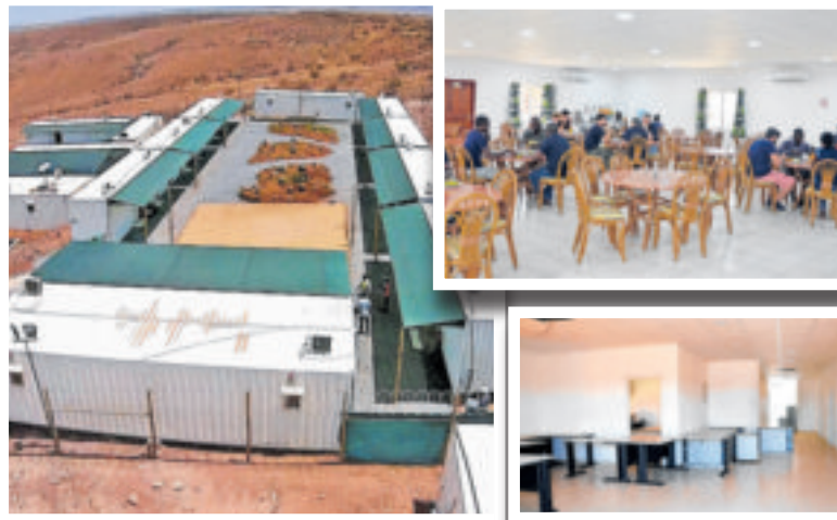
Summit camp and catering facilities. The subsidiary of Southern Engineering Company has been offering catering and accommodation services to contractors in remote areas. COURTESY
