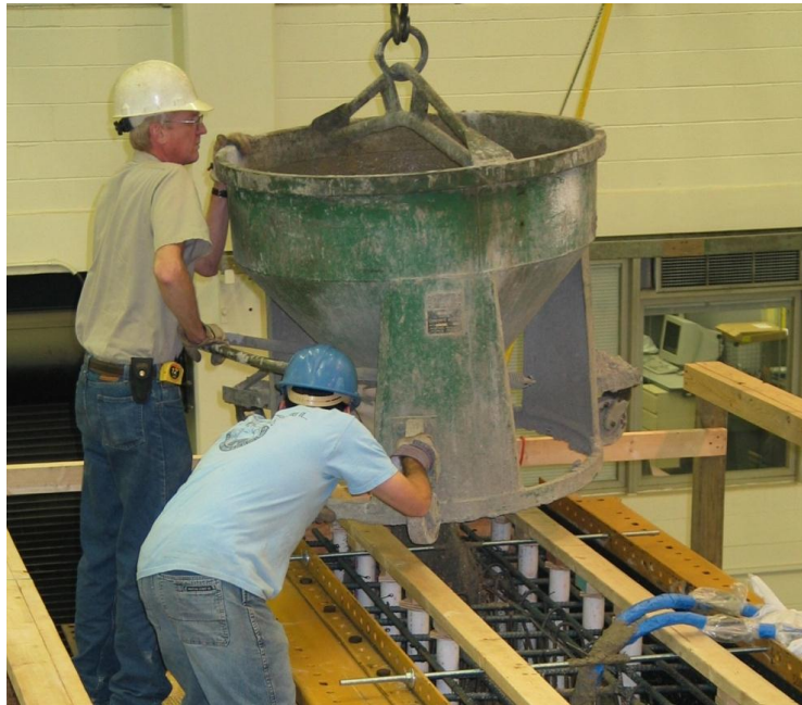
Figure 2-8: Casting a typical pier cap
