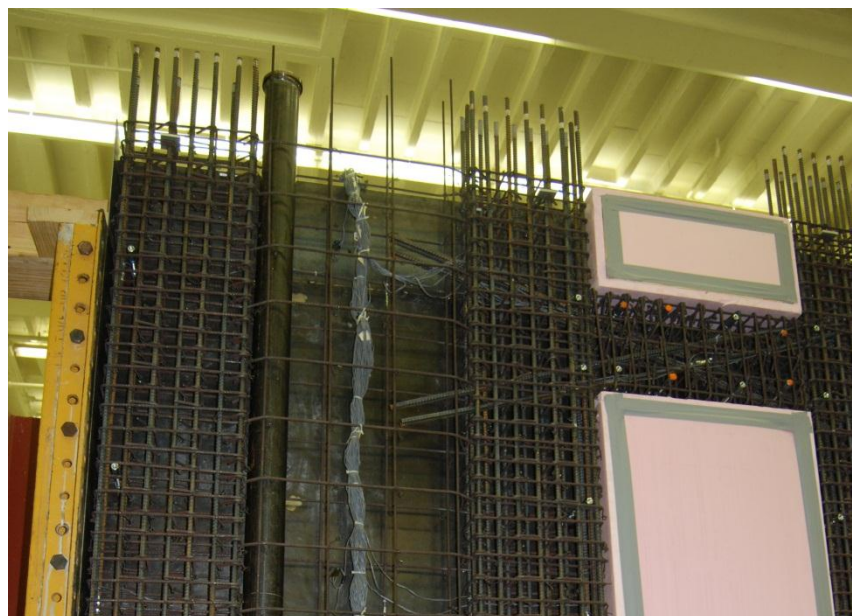
Figure 2-6: CW1 prior to casting (black steel tube 16 inches in from the left-most reinforcement)
