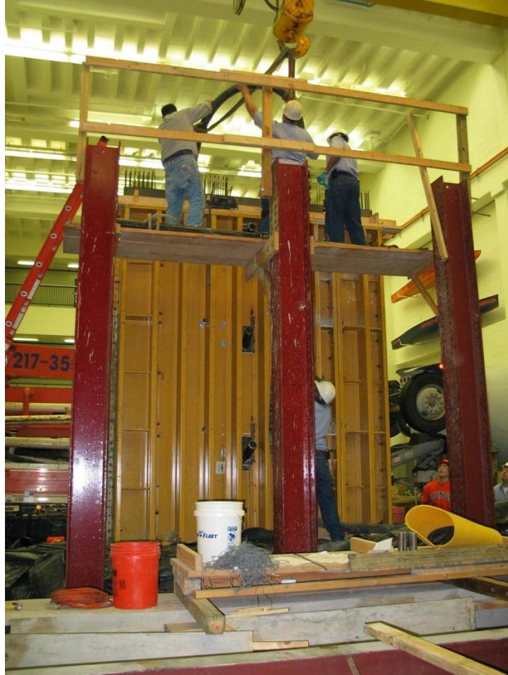
Figure 2-7: Casting of specimen via a concrete pump truck
