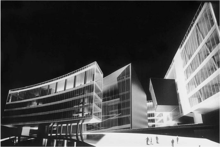
13.02 Cardiff Bay Opera House: view. © Zaha Hadid.
