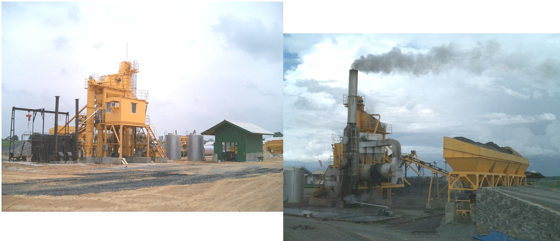
Gambar 10. 1 : Asphalt Mixing Plant.
