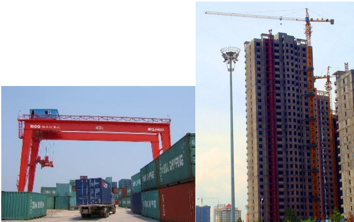
Gambar 7.3 : Rail Mounted Crane dan Tied-in Tower Crane
