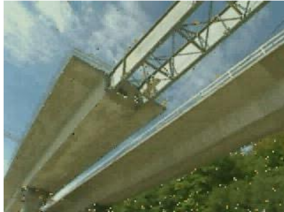
Inc. Launching Construction
