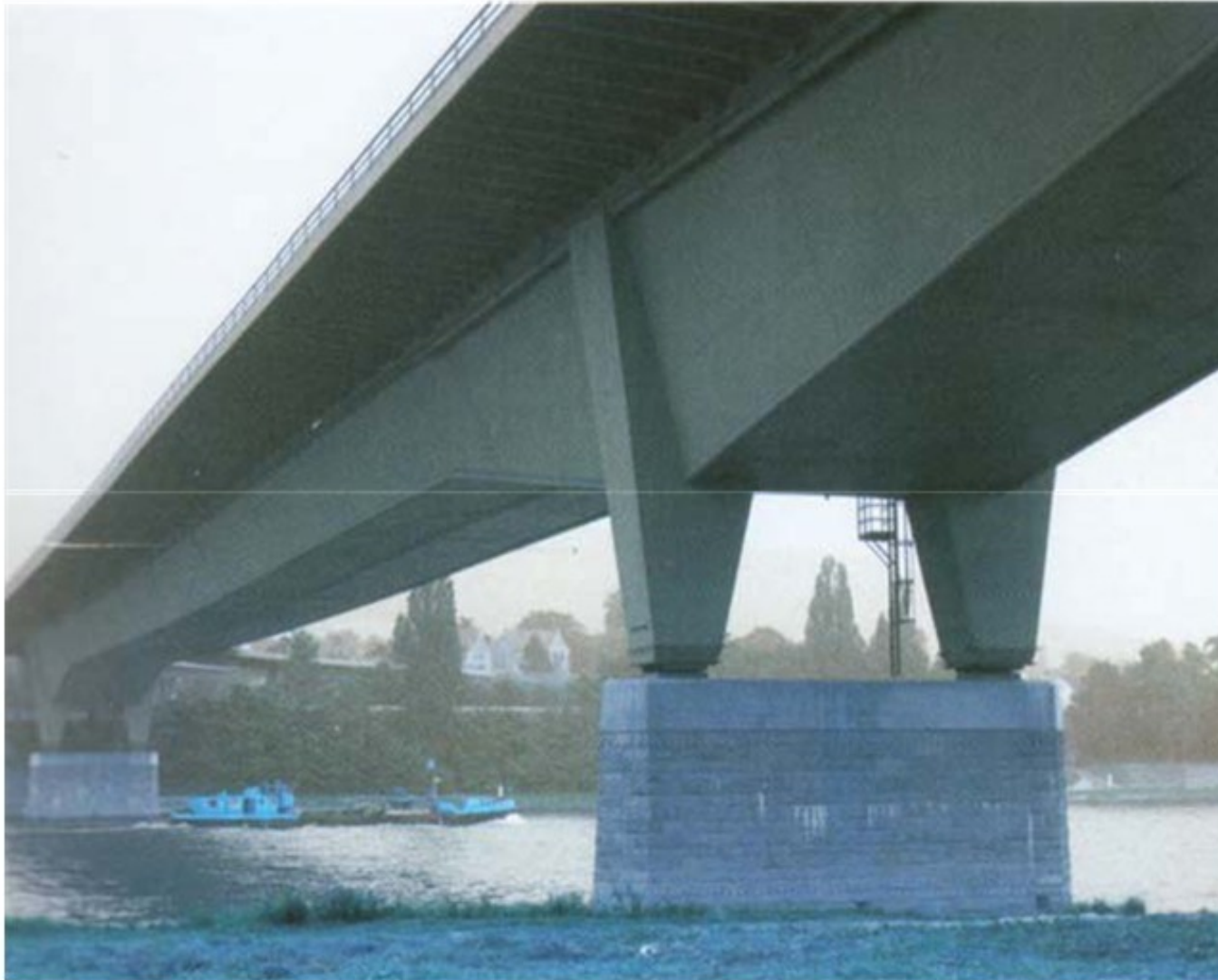
Steel Box Girder Bridge
