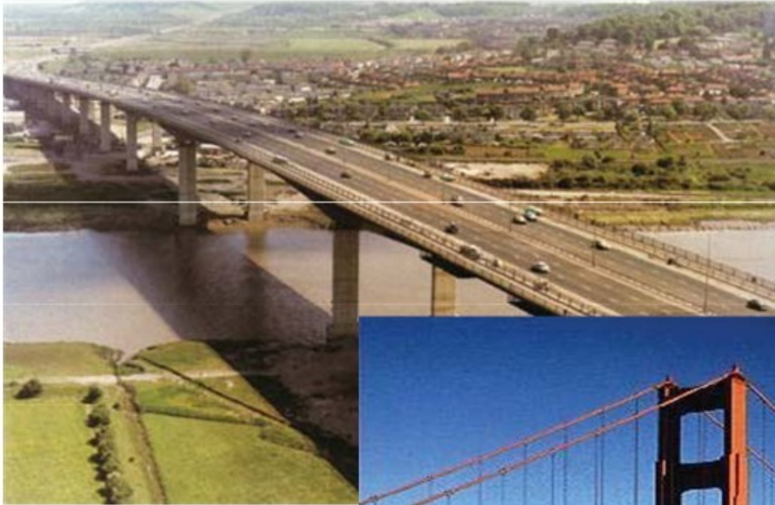
Avon Mouth Bridge Bristol, UK
