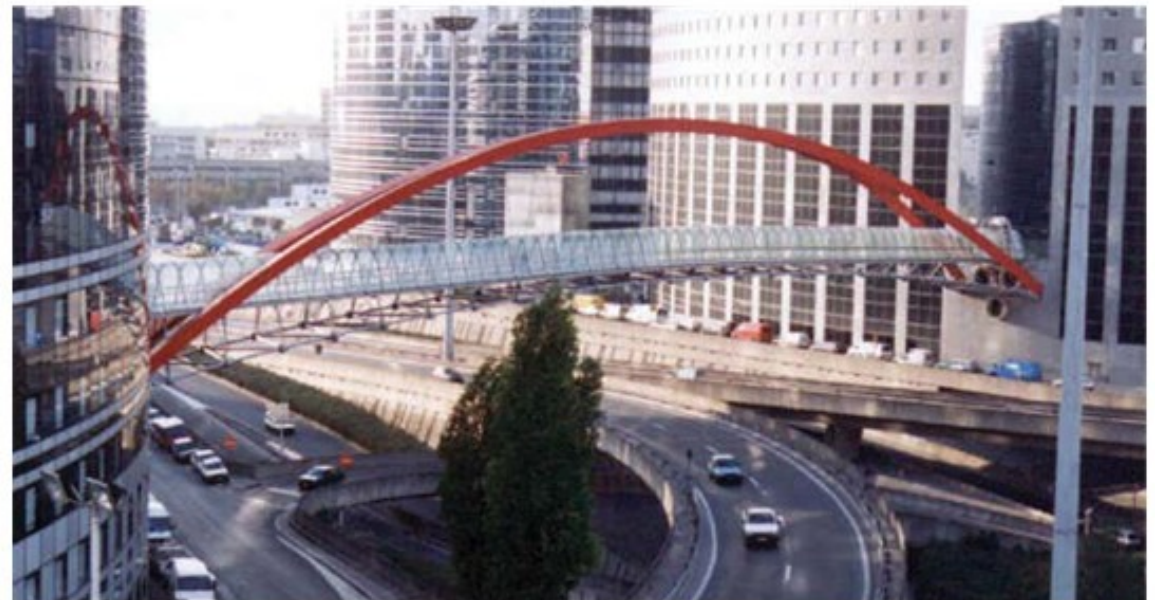
Japan Bridge (1994) Paris, France 100m span
