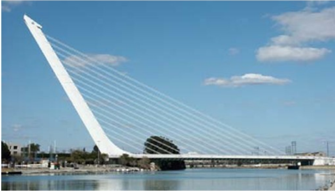
El Alamillo Bridge Seville, Spain 200m span
