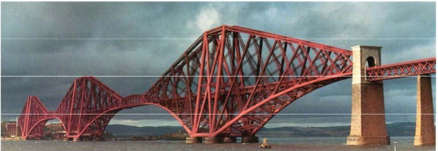
Firth of Forth Bridge (1890) Scotland 521m span
