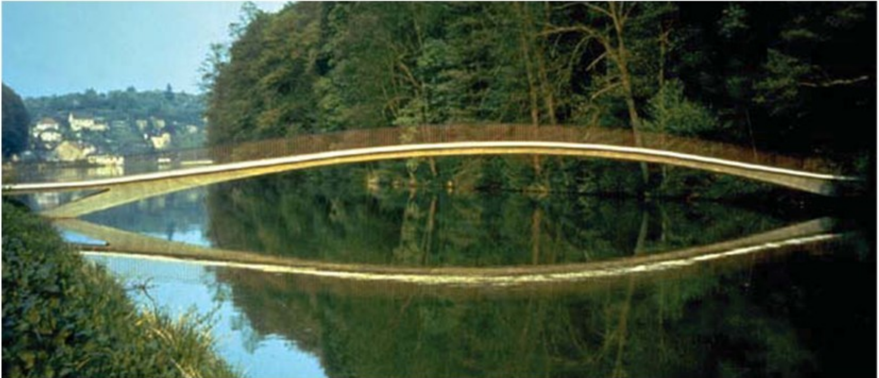
Enz Bridge (1961) Mülacker, Germany 46 m span Concrete arch
