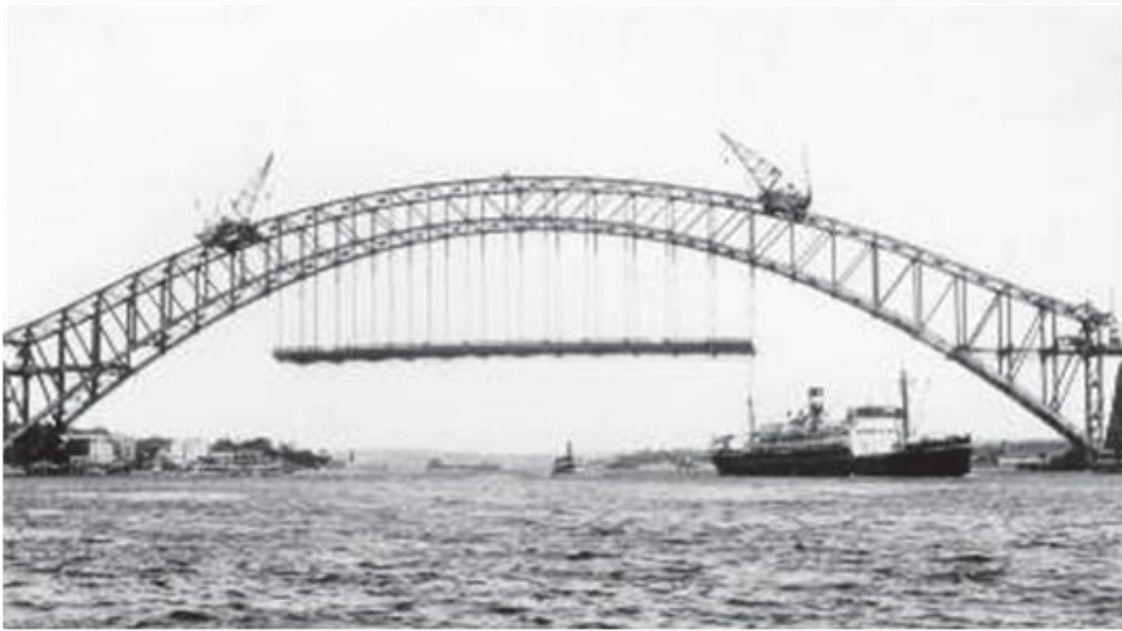
Construction of Sydney Harbor Bridge
