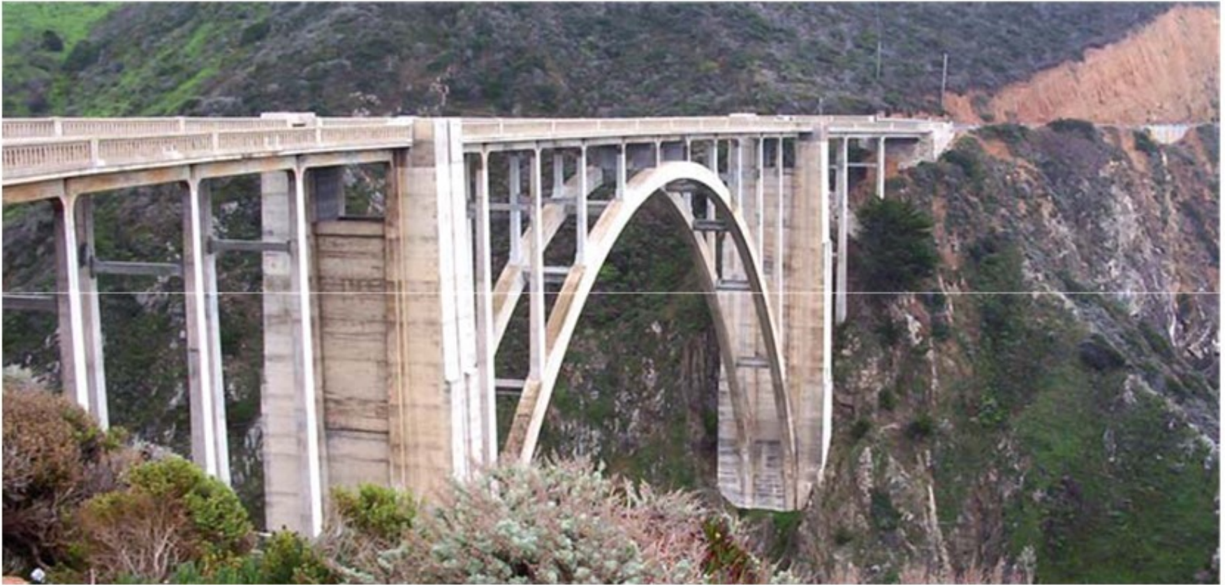
Bixby Bridge (1932) California, USA 97.5 m span Concrete arch
