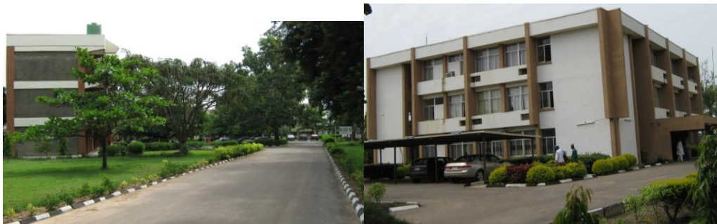
NAERLS Administrative block and a drive within.
