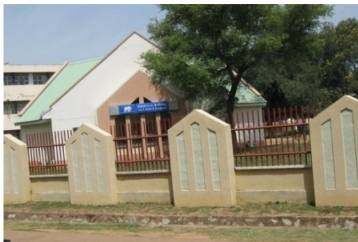
The First Bank IT Park on the Main Campus.
