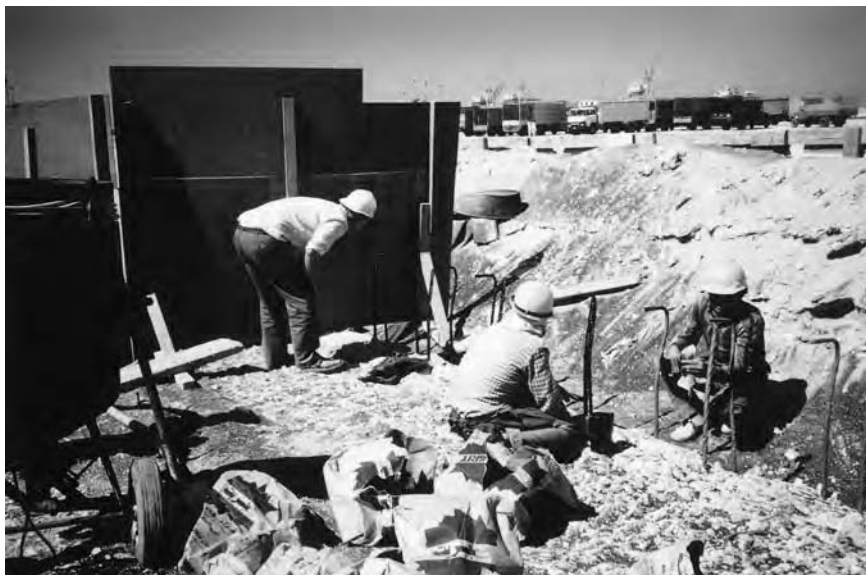
3.44 Cleaning and coating of concrete in ramp walls during repair of the Deira-Al Shindagha tunnel in Dubai.
