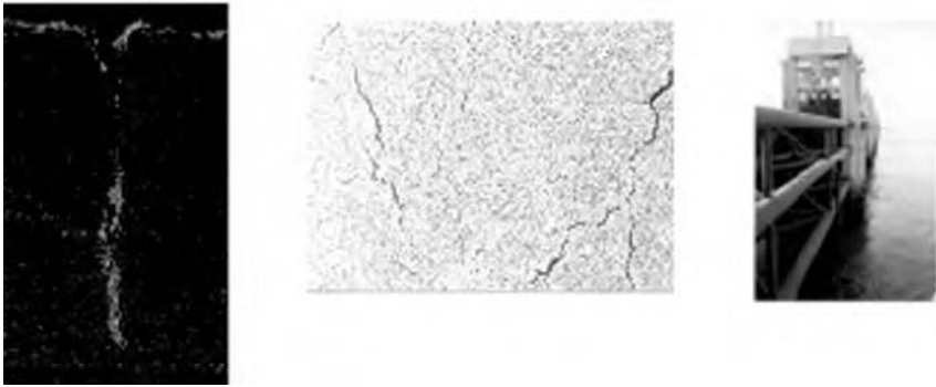
2.22 Cracks in high solids epoxy coating of Eastern Scheldt barrier in the Netherlands beneath which pit corrosion is present.
