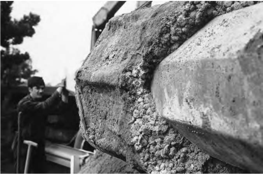
3.6 Photograph of deteriorated lamppost. 1
